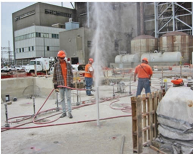
Figure 7. Blowing hole free of water prior to injection.
