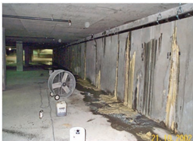
Figure 9. Urethane injection; defects are intercepted at depth and grout returns to surface can be quite messy.
