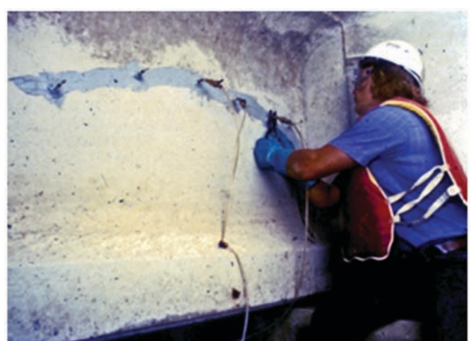
Figure 8. Typical epoxy injection from surface. Cracks are pre-sealed and operation can be quite neat.
