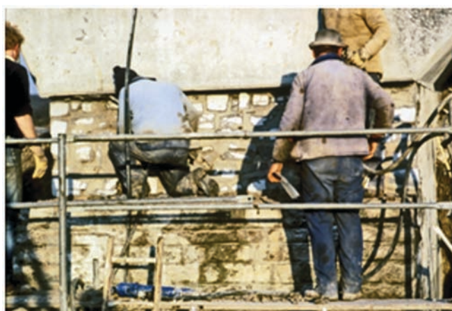
Figure 12. It is good practice to repoint and seal masonry surfaces prior to injection.
