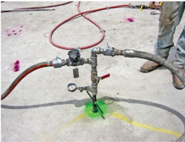
Figure 5. Typical grouting header for circulating injection system. Supply hose on right, return on left. Valve above gauge controls injection rate.
