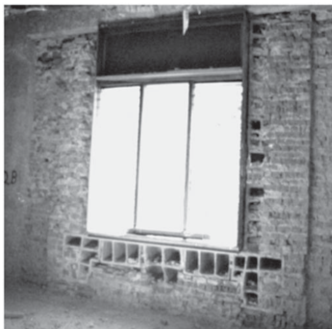
Figure 10. Large and sometimes continuous voids are common in older masonry.
