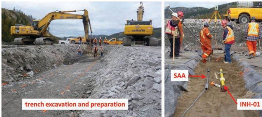
Figure 3. Installation of INH-01 and SAA.
