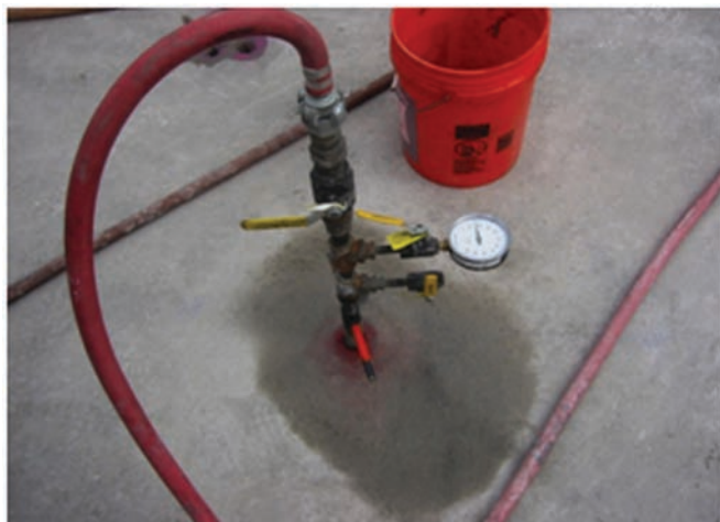
Figure 3. Pressure testing grout hole using line pressure of facility system.
