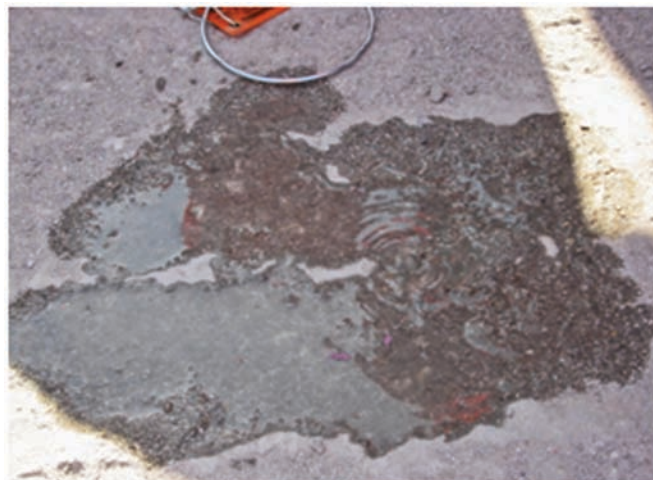
Figure 4. Leak on the surface in an area where no problem was previously visible.
