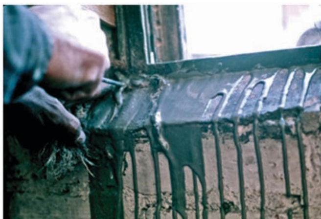
Figure 11. Grout leakage is usually a huge problem when injecting grout into masonry.
