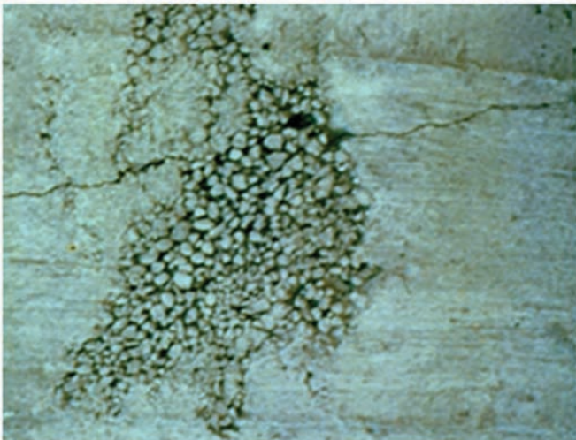
Figure 1. Here are two defects in one location. Both honeycomb and a crack are visible.
