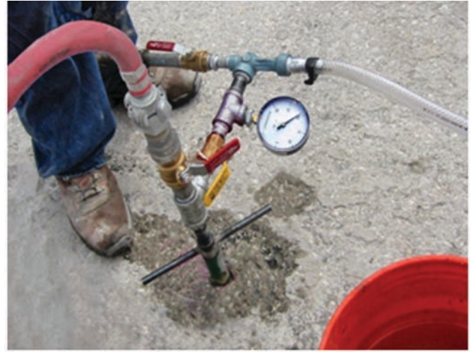
Figure 6. Vacuum grouting header. Valved hose top left is compressed air entering venturi ejector, white hose on right carries away spent air. Upon sufficient vacuum, valves are turned from vacuum to grout.
