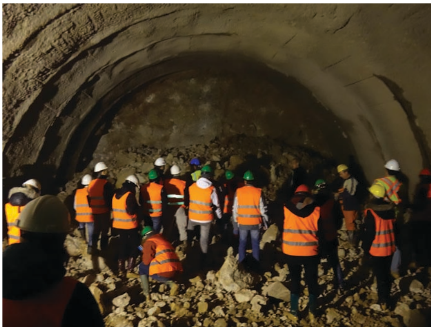
Crystallogipi Tunnel: conventional tunnelling students viewing the tunnel face minutes after explosives were detonated.
