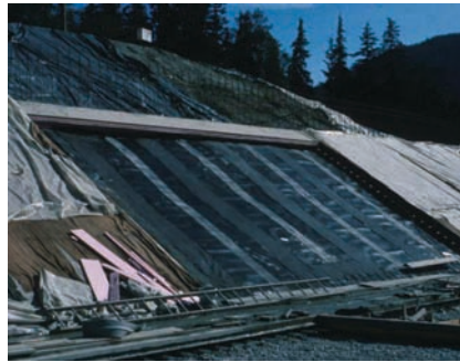
Figure 1b. Inclined sidewall of the spillway channel.
