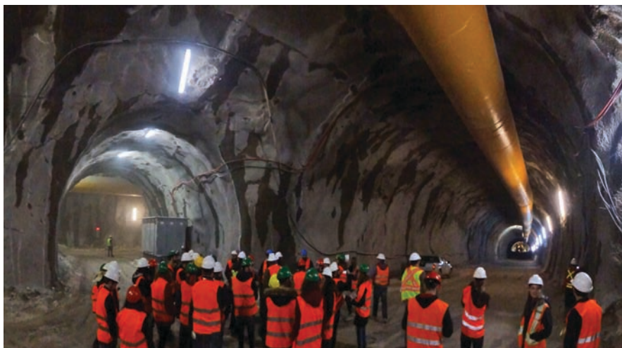
Klokova Tunnel (Ionian Odos): conventional tunnelling – heading and bench - course visit.
