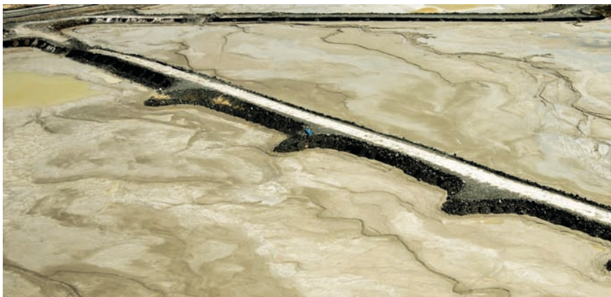
Waste rock inclusion constructed in the tailings impoundment at the Canadian Malartic mine. Such inclusions act as drainage and reinforcement elements to improve the hydro-geotechnical behaviour of the impoundment (photo provided by Osisko).
