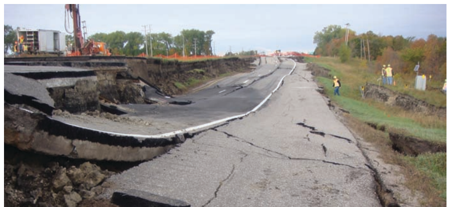
Figure 2. SAA systems reported and recorded a significant landslide event in near-real-time to geotechnical offices five hours away. The SAA systems remained fully operational as over 100 inches (2.5 m) of lateral deformation was measured.
