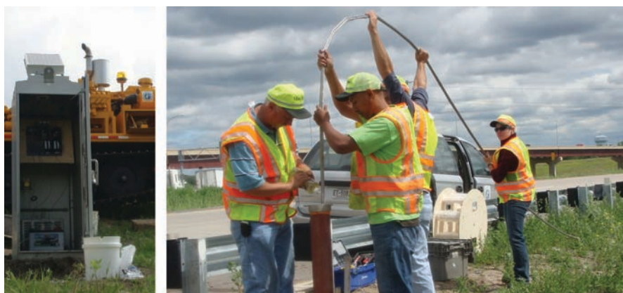
Figure 1. Typical SAA up-hole cabinet (left) and crew installing a SAA sensor in a borehole (right).
