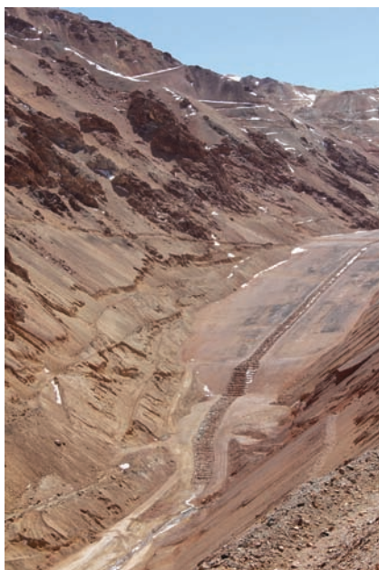
Photo 3. The closed and covered tailings at El Indio, Barrick's pioneering work that set the national reference point for mine closure practice in Chile. Photo shows the closed and covered tailings deposit in the valley, with channel restoration along the axis of the deposit.
