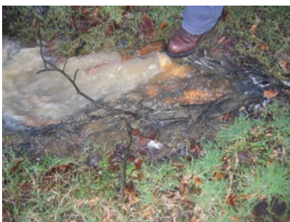
Figure 1. Seepage evidence at the Carno dam.
