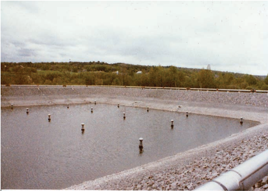
Figure 1. Example of half-full lagoon for wastewater treatment (photo by author). The pipe (bottom right and along the crest of the dike) provides air to the aerators, the upper part of which emerges in the partially filled lagoon. Two influent or effluent pipes can be seen above the water line.
