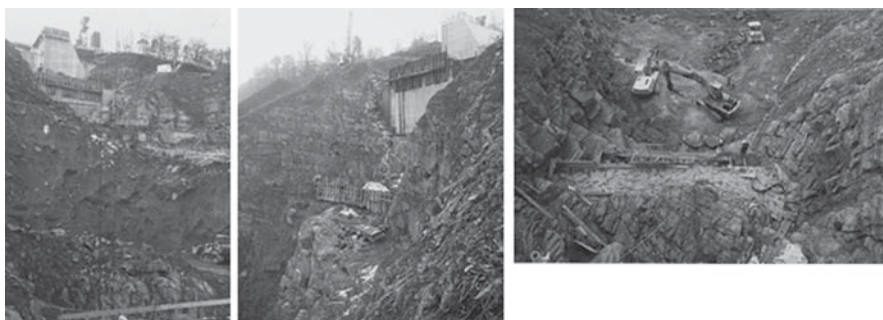
Figure 1. Wimbleball Dam foundation excavation.
