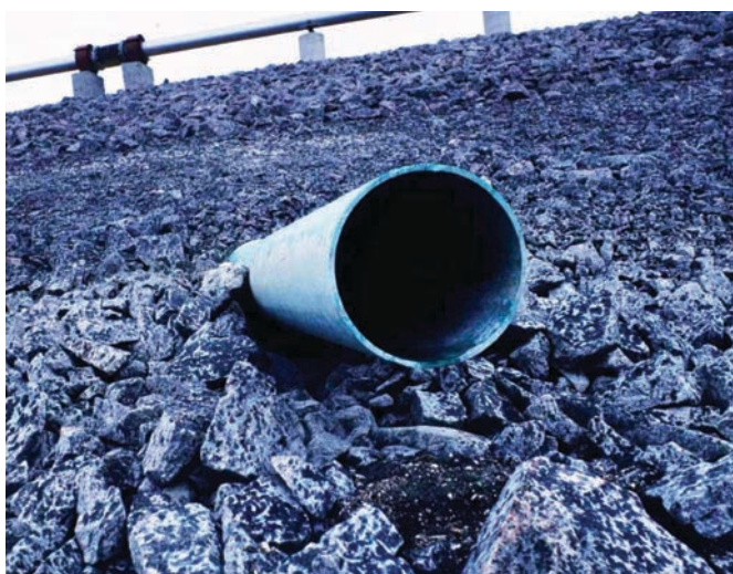
Figure 4. Photograph of the poor contact between a pipe and the clay liner (photo by author). A large opening appears as a black crescent below the pipe.
