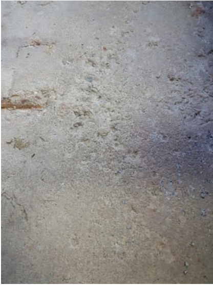
Figure 1. Shows a poor surface for reflectorless monitoring.
