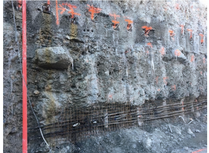
Figure 11: A bouldery frozen area in during winter excavation
