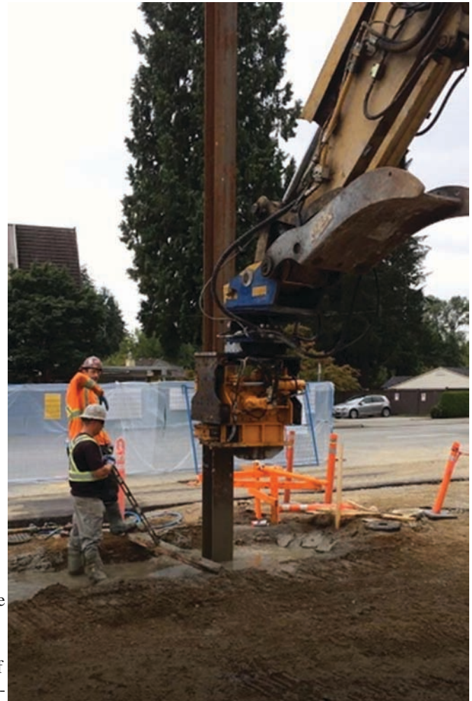
Figure 6: H beam installation with vibrator.
