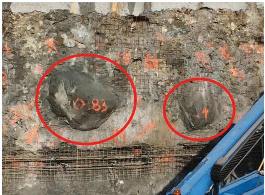
Figure 7: Excavated north wall with boulders Figure 7.jpg
