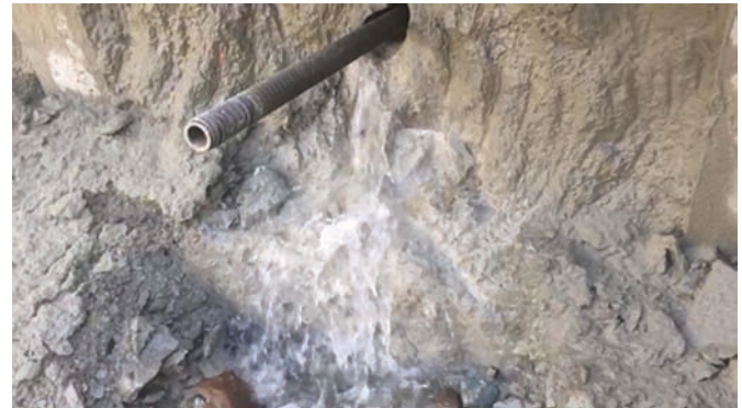
Figure 12: Water from the drilled soil anchors.
