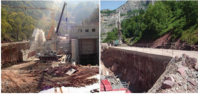
Figure 9: On the left - Works in progress with the jet grouting wall protection from the river bed.
