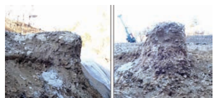
Figure 8: Jet grouting trial columns executed at the start of the works.
