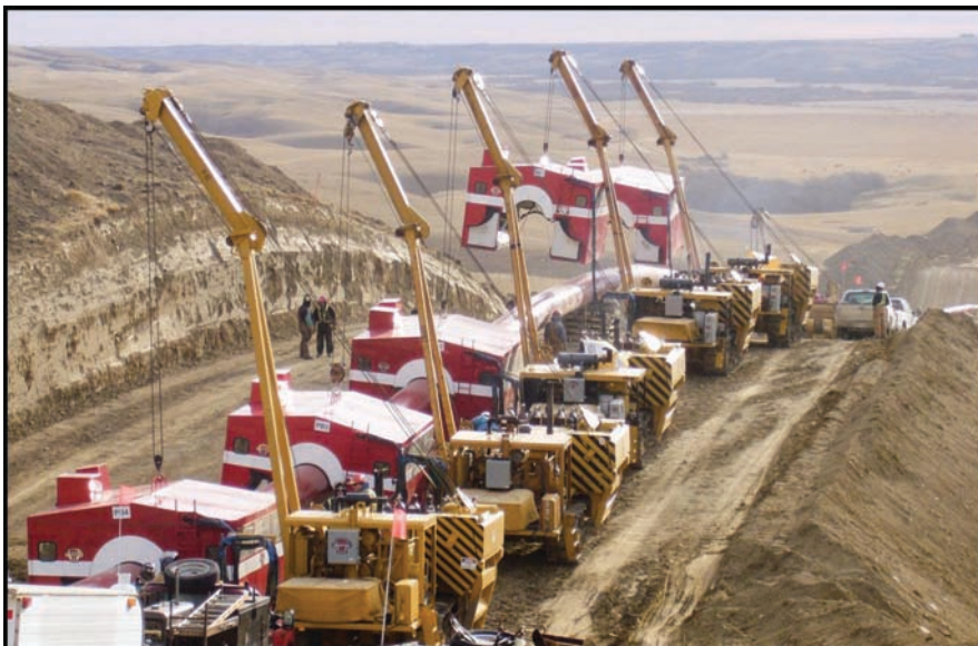
Figure 3: A large-diameter pipeline under construction (photo ©Tim Bossenberry, used by permission).
