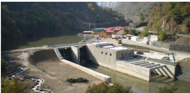
Figure 1: Power plant of Lakatnik.
