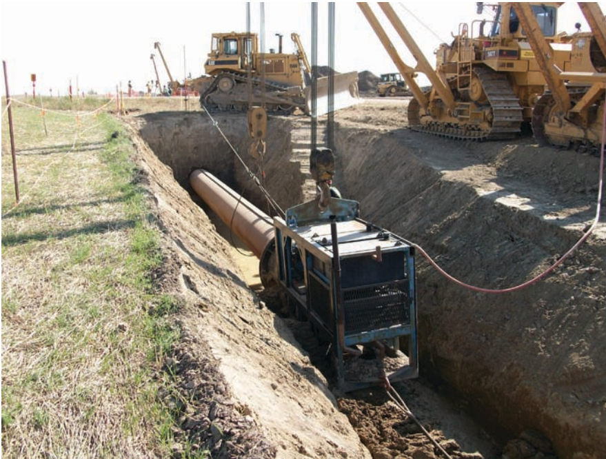
Figure 4: Cradle boring setup (Image ©Mike Wagner, used by permission).
