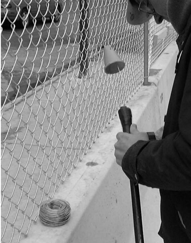
Figure 8. View of the sealed end tip of a flexible TDR sensor cable also fitted with a plastic cone to catch the PVC grout tube for insertion
