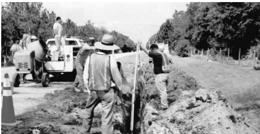
Figure 1. Installation of horizontal TDR sensor cable in a grouted trench over a stabilized sinkhole
