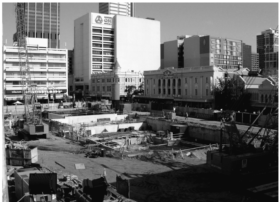
Figure 4. Buildings being monitored around the William Street Station Box in Perth, Western Australia.
