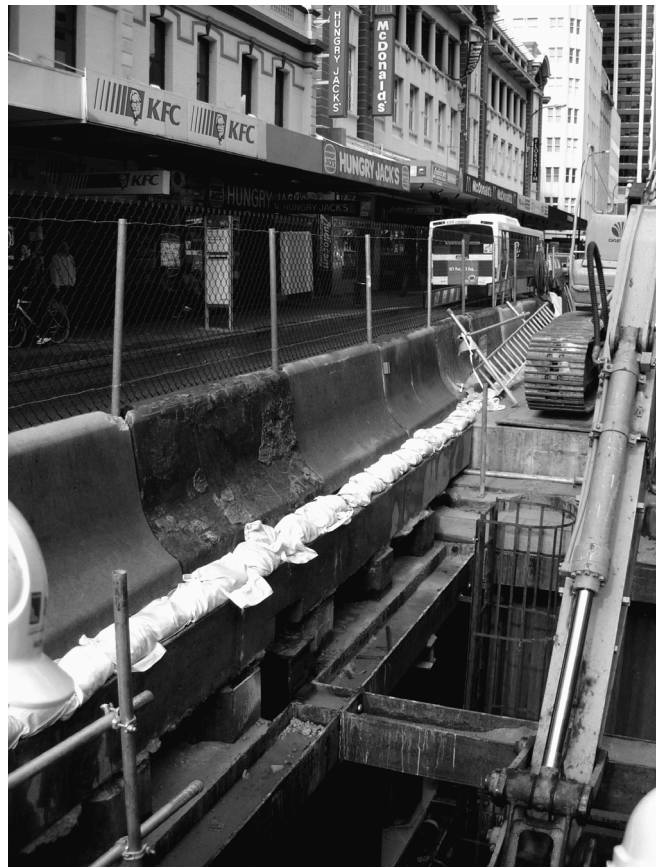
Figure 6. Excavation in Perth and buildings being monitored.
