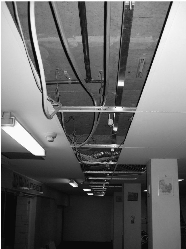
Figure 5. Radio EL beams installed above a false ceiling.
