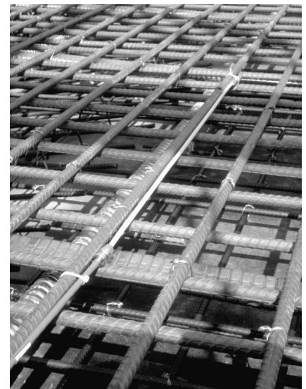
Figure 5. SOFO sensor installed on a rebar. The plastic pipe contains the coupled measurement fiber and a free un-coupled reference fiber. The metallic anchors at both ends of the white plastic pipe define the gage length.
