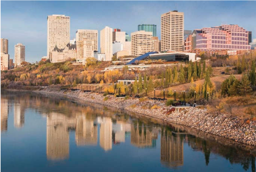
Shaw Convention Centre, Edmonton, Alberta.
