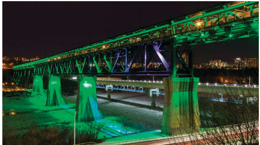
High Level & LRT Bridges, Edmonton, Alberta.
