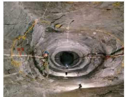
Examining excavation stability in rock having high differential stresses.
