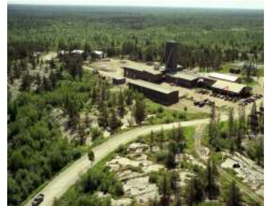
Atomic Energy of Canada's URL, surface facilities.
