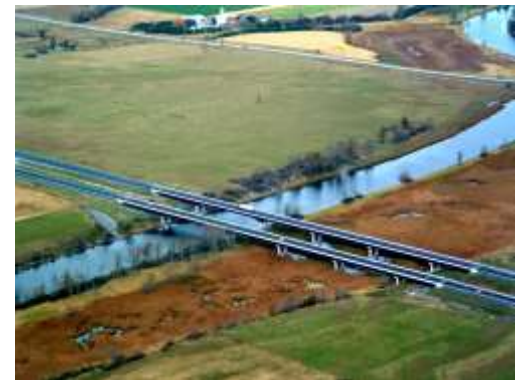
Twin Mississippi River bridges carrying Highway 417 over the Mississippi River and the adjacent wetland.
