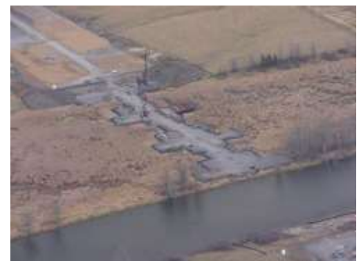
Foundation construction in wetlands.
