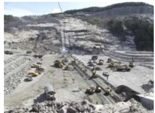
The main Romaine-2 Dam during construction.
