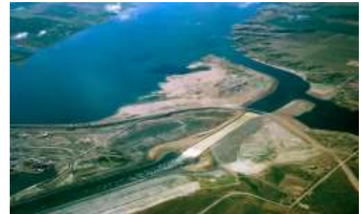
Aerial overview of the Gardiner Dam
