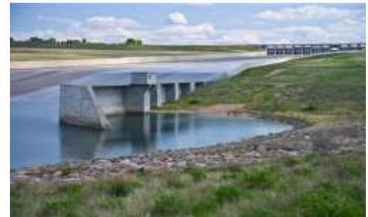
Gardiner Dam Spillway.
