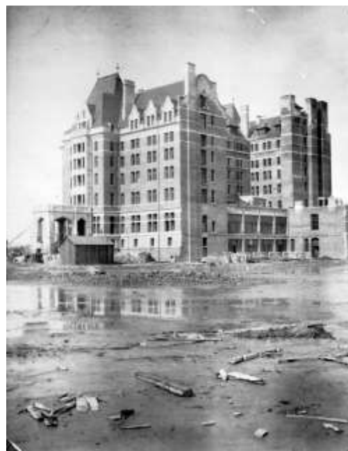
Empress Hotel nearing completion in 1907. View from the southeast overlooking a portion of the reclaimed tidal mudflat upon which much of the hotel was constructed. Image D-07275 courtesy of the Royal BC Museum and Archives.
