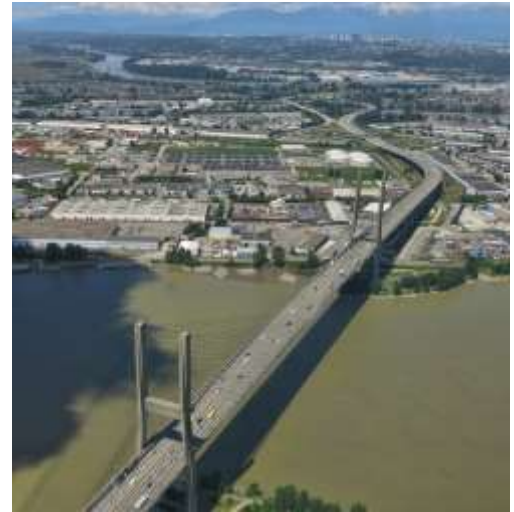
Aerial view looking north
