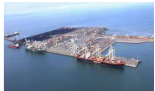
Deltaport Container Terminal looking west.
