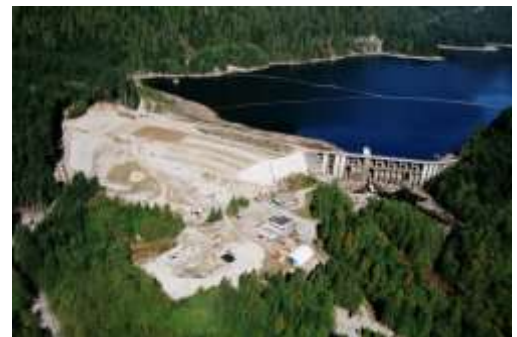
Aerial view of dam in 2006.
