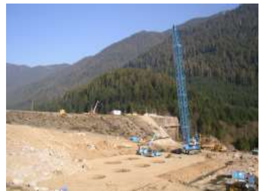
Dynamic compaction densified dam's foundation (2005).
